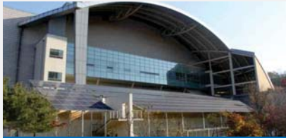
Mapo Waste Incineration Plant, PV 120 kW
