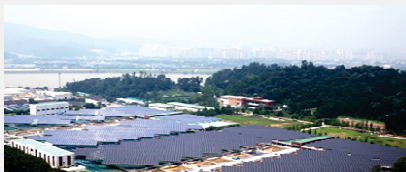
Amsa Water Plant (5,000 kW) Completed in July, 2013
